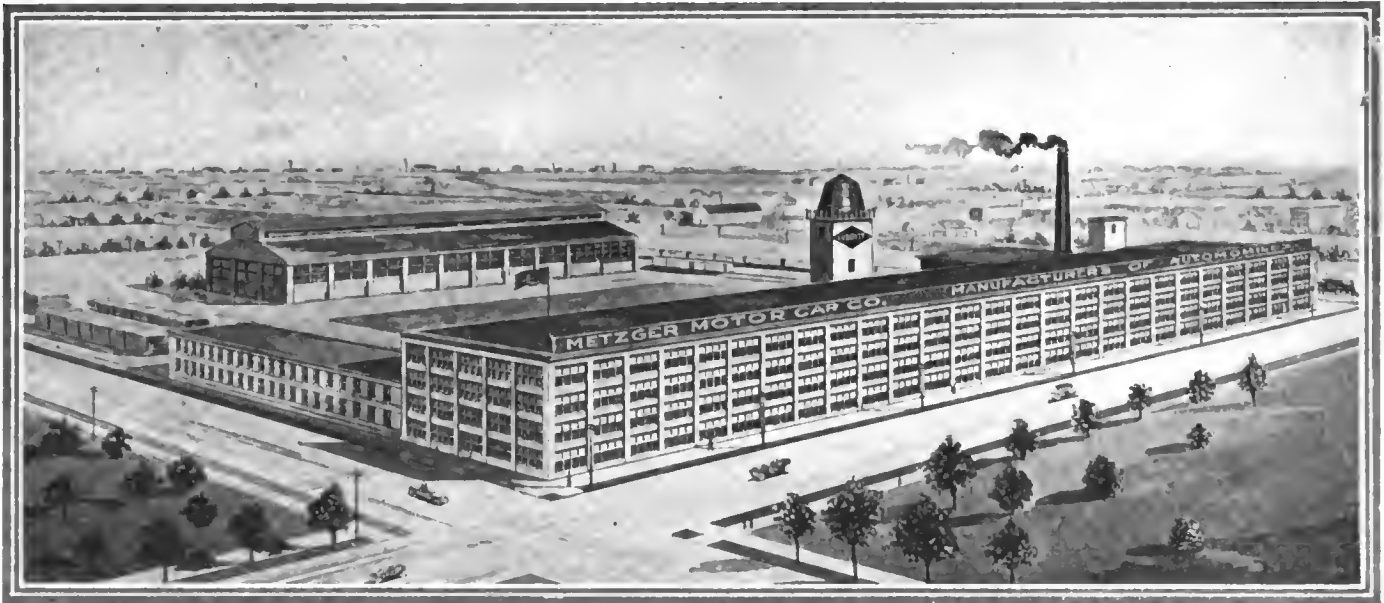
New building of the Metzger Motor Car Company, at Detroit, Mich., now in course of construction. It is four stories high and 550 feet long
